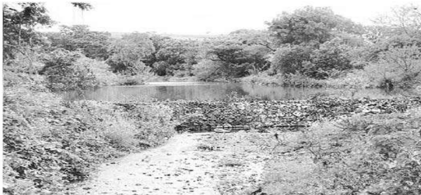
Figure 8 Gabion Weir
