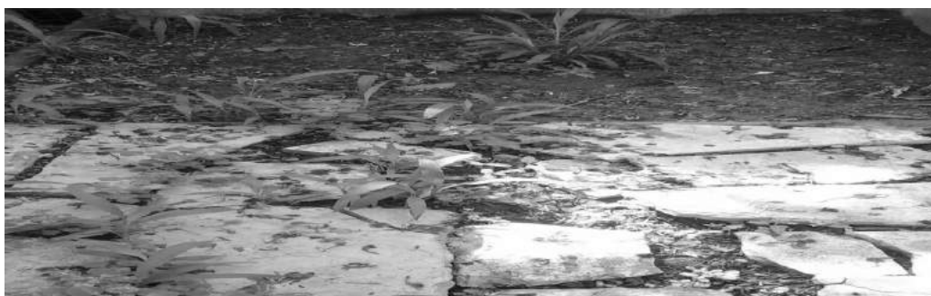
Figure 6 Unpaved Area adjacent to the Well
