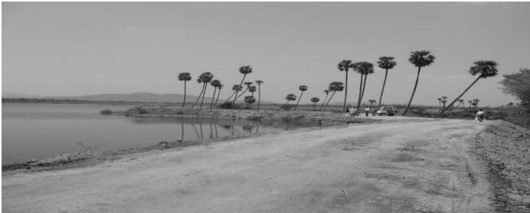
Figure 7 De Silted Tank
