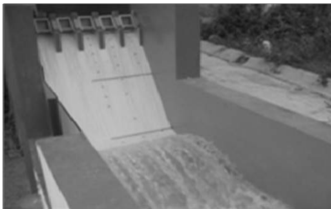
Figure 2. Photograph of Provision of air vent of dia 0.02 m
