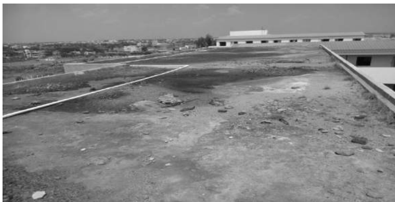
Roof of BIET Main block
