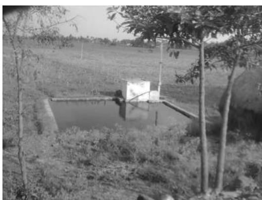
Figure 8 Dug well at Lathuvadi
