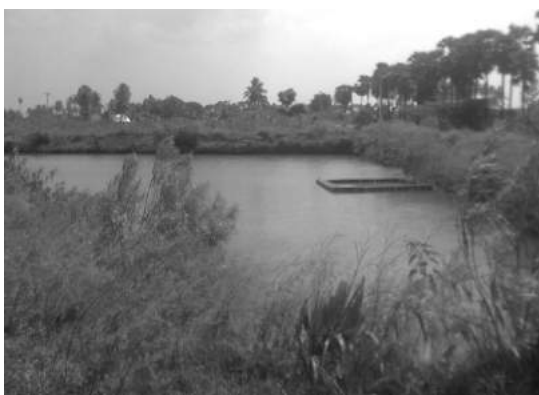
Figure 6 Percolation pond with recharge bore well, Lathuvadi
