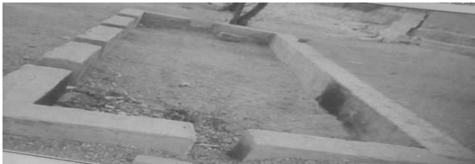
Figure 4 Water Harvesting Structure
