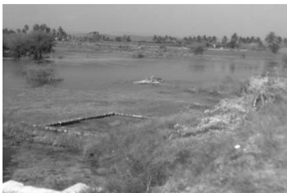
Figure 7 Desilted village pond with recharge bore well, Veeraganur
